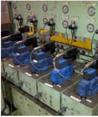
Eaton's Vickers KBHDG5V-7 Series two-stage, servo-proportional directional valves provide accurate high speed profiling on valve stands.
